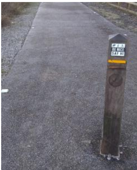
Plate 7.1-Brittania Greenway Nu-flex section in sub-zero temperatures showing no ice
